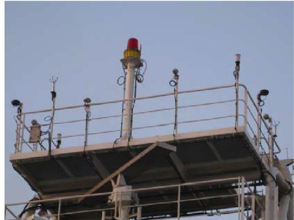
Good antenna location
